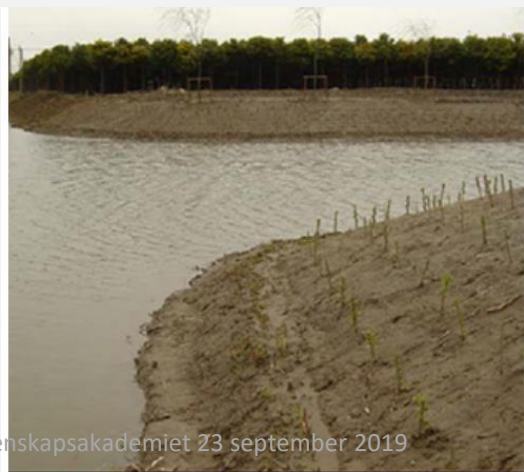
Figure 1. Live staking on the riverbanks of the Airport Town, Shanghai. In the left picture: 10 days after the installation, in the right picture: 140 days after the installation.
